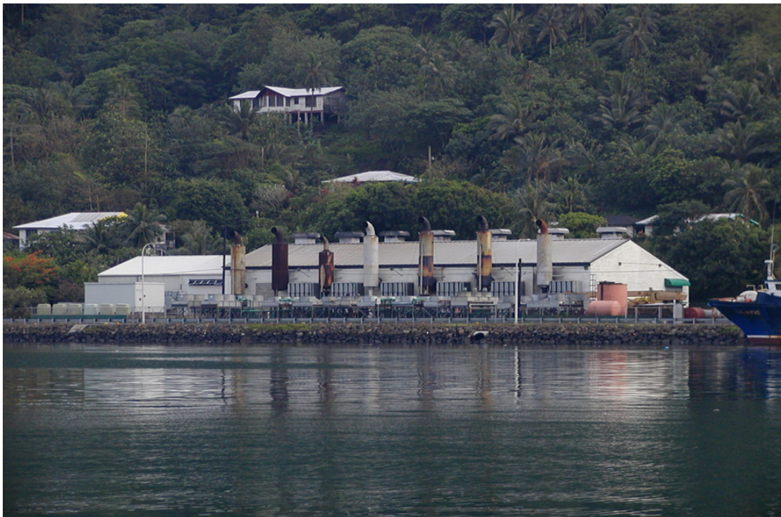
Figure 4. The Satala Power Plant, Tutuila, American Samoa prior to an earthquake and tsunami
