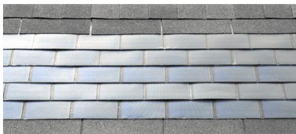
Figure 19. Thin film solar PV shingles
