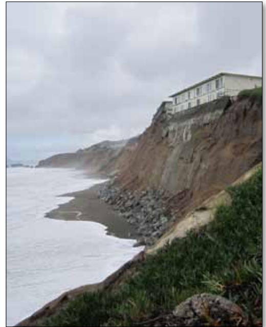
Houses near the edge of a rapidly eroding section of cliff in Pacifica, CA., illustrate the risk that sea cliff erosion poses to residences and infrastructure in many locations along the U.S. West Coast. Photo credit: Gary Griggs, Univ. of California-Santa Cruz
