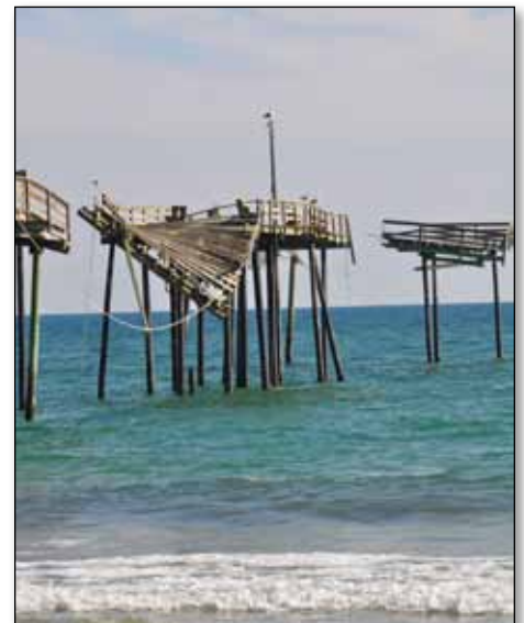
A pier on Cape Hatteras battered by waves and surge associated with extreme storms. Photo credit: Ann Tihansky, DOI.
