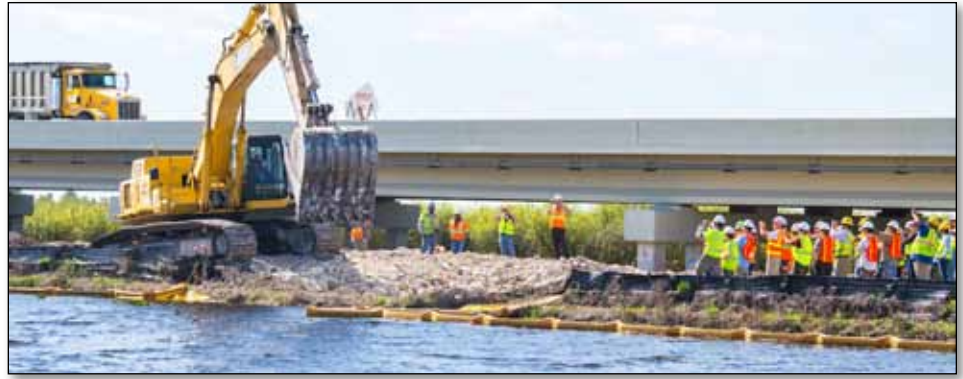
Construction crews restore flow to a part of the Everglades by removing a section of the Old Tamiami Trail in South Florida. Photo credit: NPS
