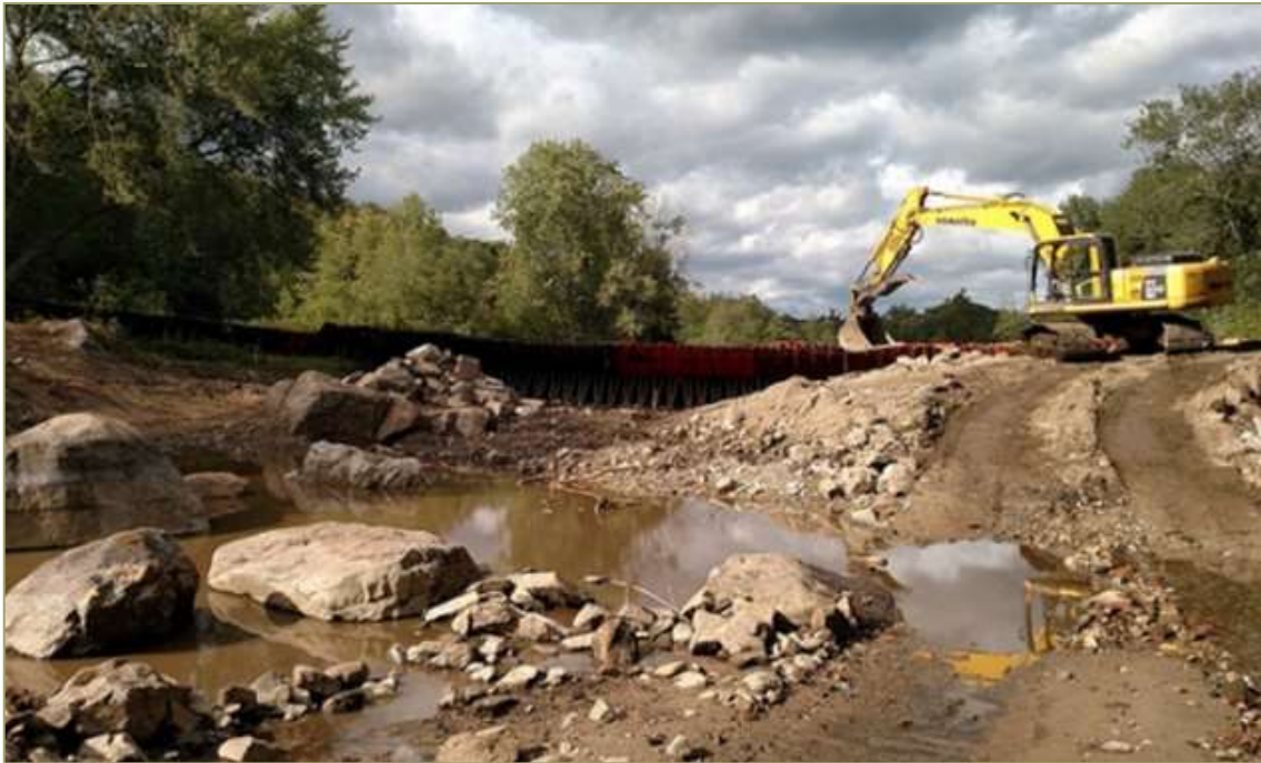
The removal of White Rock dam on the lower Pawcatuck River (Scott Comings)
