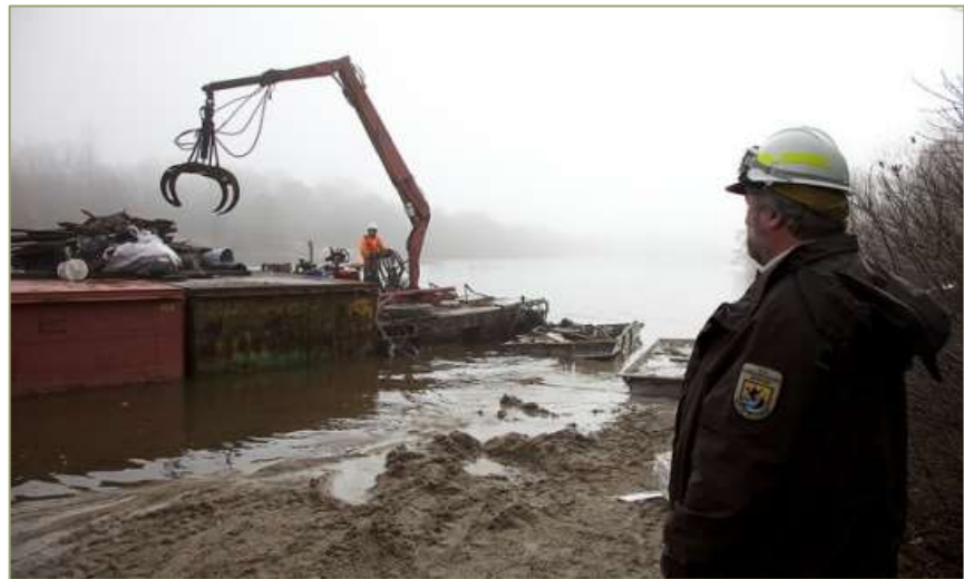
Water-based debris removal at Forsythe National Wildlife Refuge (Ryan Hager)
