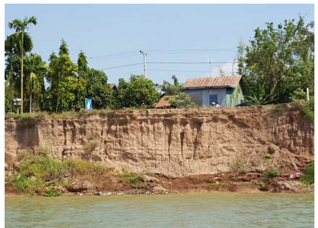
River bank erosion on the Mekong. Credit: DOI- ITAP.
