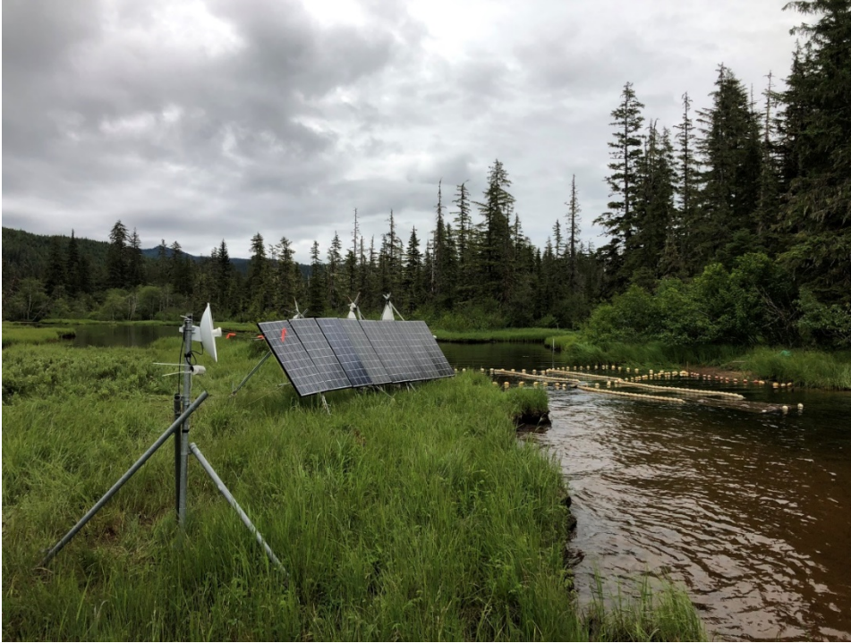
Figure 3. The video weir at the outlet of Sitkoh Lake, July 9, 2020.
