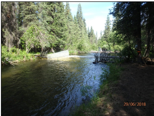
Tanada Creek fish weir
