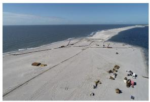
million cubic yards of OCS sediment was used to fill the 2.4 mile-wide Camille Cut during the first phase of the project in 2018-2019. Filling the breach is part of a long-term commitment to improve the health and ecosystem of Mississippi Sound.
