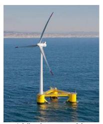
A full-scale prototype of the WindFloat device
