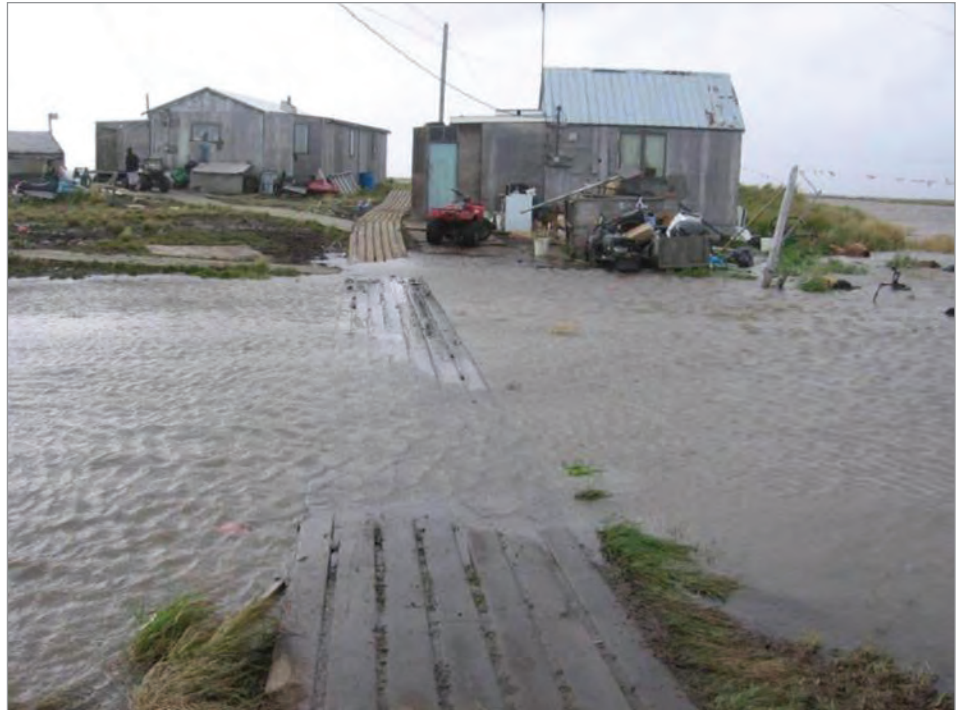
Flooding in the village of Newtok during the 2005 Fall Sea Storm. Photo credit: Stanley Tom, Newtok Traditional Council
