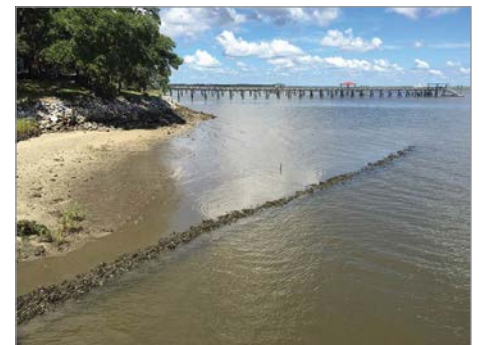
South Carolina Coastal Program built oyster reef providing erosion control for property in Beaufort County. Photo credit: USFWS
