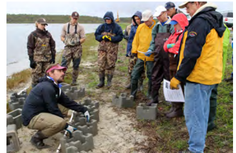
Volunteers assemble oyster castles to create an oyster reef living shoreline at Chincoteague National Wildlife Refuge. Credit: Chelsi Burns, USFWS
