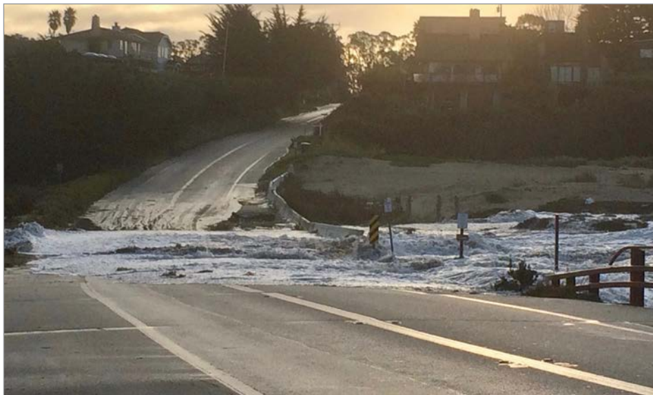
Waves flood across a coastal road near Santa Cruz, CA. Photo credit: Amy Foxgrover, USGS
