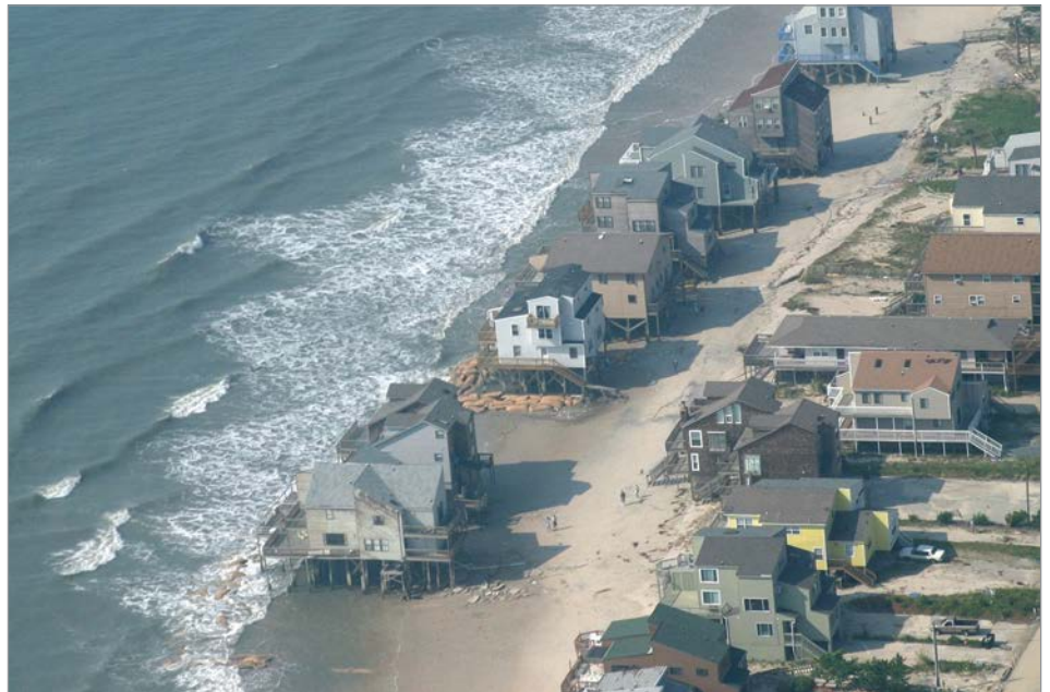
Aerial view of North Topsail Beach, NC, showing homes in the surf after Hurricane Ophelia. Photo credit: Program for the Study of Developed Shorelines, Western Carolina University
