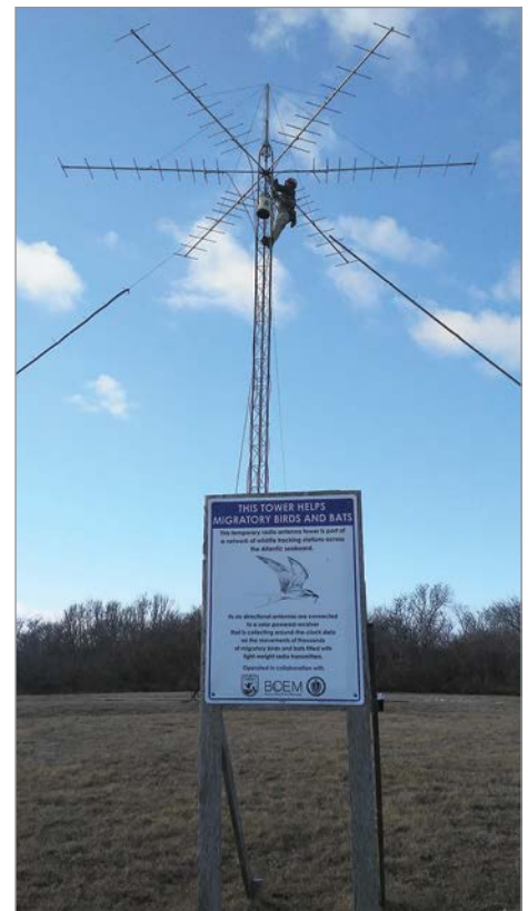
Brett Still assembling an antenna used for tracking tagged birds on Block Island, RI. Photo credit: Pamela Loring, USFWS
