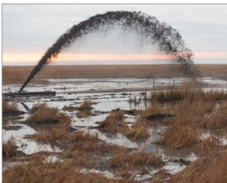
Sediment is sprayed onto a marsh at Blackwater National Wildlife Refuge, MD, to compensate for its natural tendency to sink and the effects of sea-level rise. Photo credit: Dave Harp, Chesapeake Photos
