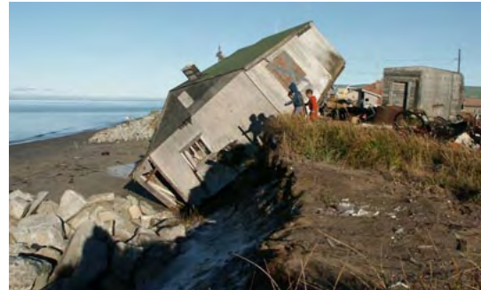
As permafrost thaws, the ground under a home in Shishmaref, Alaska collapses from erosion.
