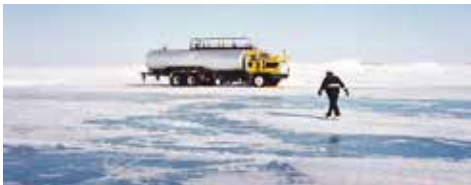
Construction of ice roads is crucial for Alaskan North Slope operators to gain access for exploration in an economic and environmentally sound manner. Photo: DOE
