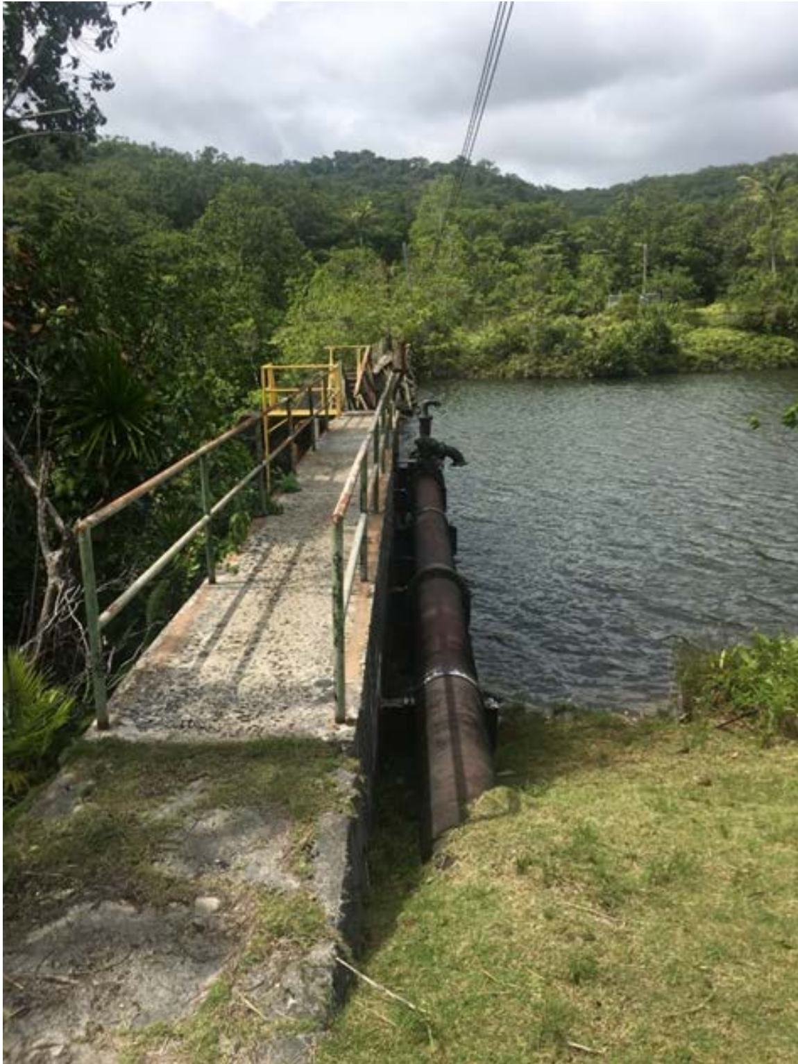
Figure 11.—The Ngerimel Dam and Reservoir.
