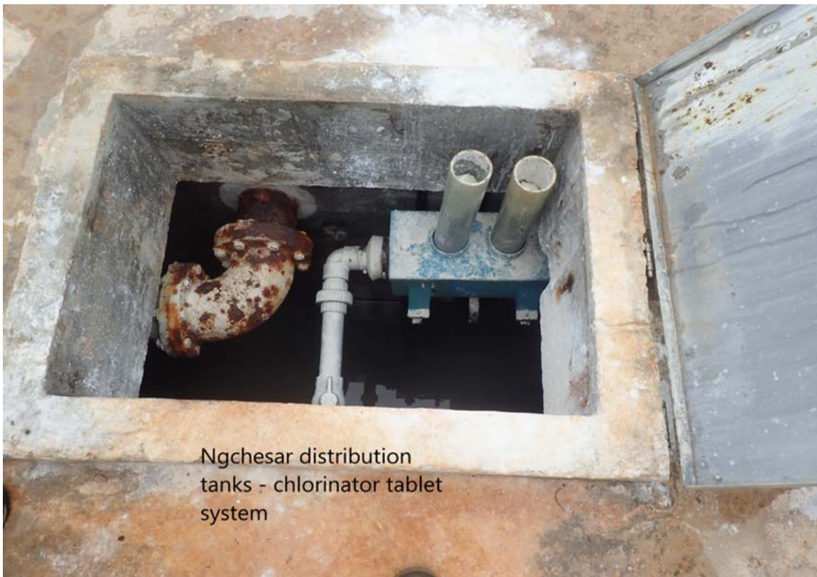
Figure 8.—Three-inch chlorination tablets stacked within plastic tubes at the Ngchesar plant clearwell.
