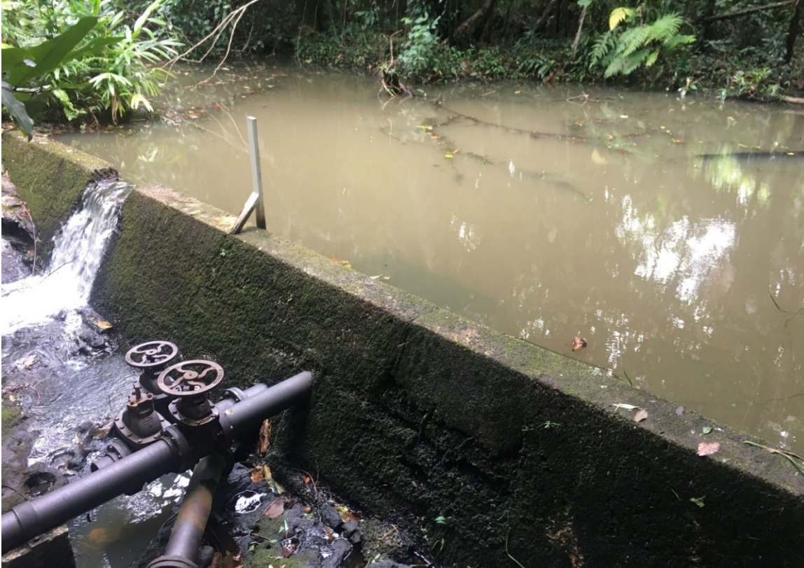
Figure 2.—The Aimeliik Ngchemiangel dam and intake system.
