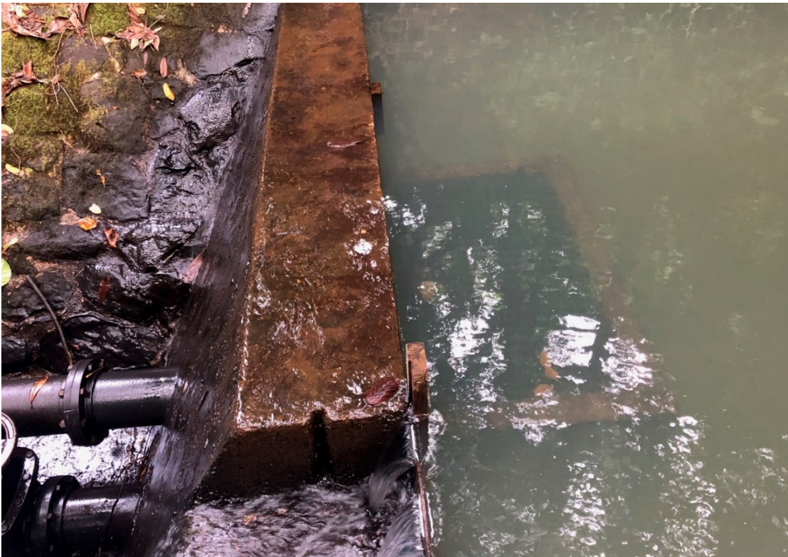
Figure 3.—The Ngaraard Ulimang dam and intake system.
