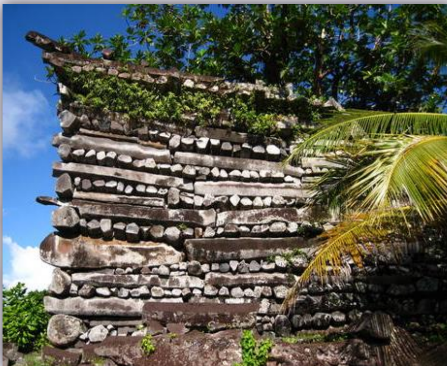
Description: Nan Madol: Ceremonial Center of the Eastern Micronesia: Columnar basalt used in a wall built by in a header-stretcher technique Nandowas Isle Date: 01/01/2012 Author: Takuya Nagaoka
