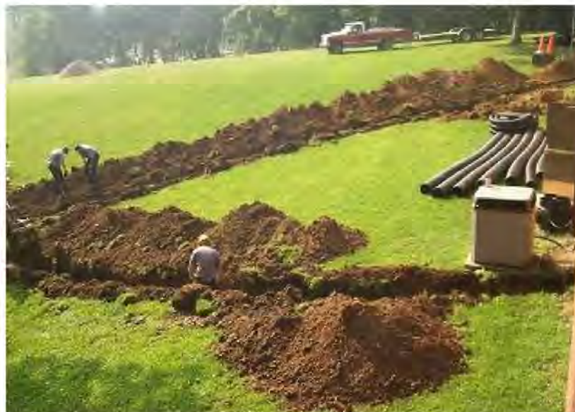
Park headquarters drainage improvements (2000) performed without completing Section 106 review. Geophysical evidence now shows many mound remnants – potentially with intact burials – in the headquarters vicinity. NPS photo.
