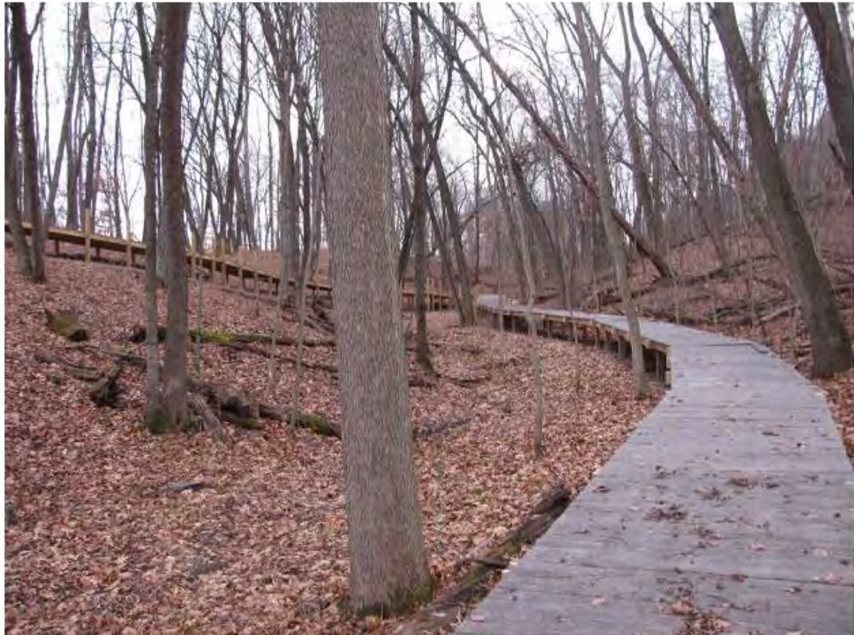
Nazekaw Terrace Boardwalk, constructed without completing SHPO or tribal consultation in 2008-09 (construction terminated by the NPS in 2009, boardwalk removed in 2010). NPS Photo.
