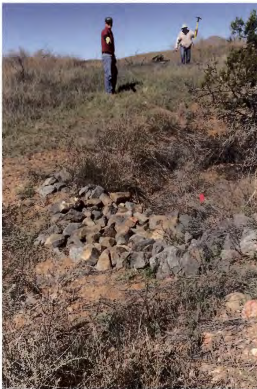
A volunteer points out a section of a breached check dam.
