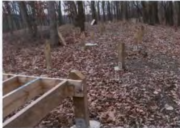
Nazekaw Terrace Boardwalk construction terminus (linear mounds visible in left background). NPS Photo.
