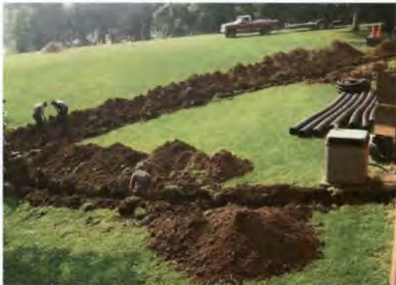
Park headquarters drainage improvements (2000) performed without completing Section 106 review. Geophysical evidence now shows many mound remnants – potentially with intact burials – in the headquarters vicinity. NPS photo.
