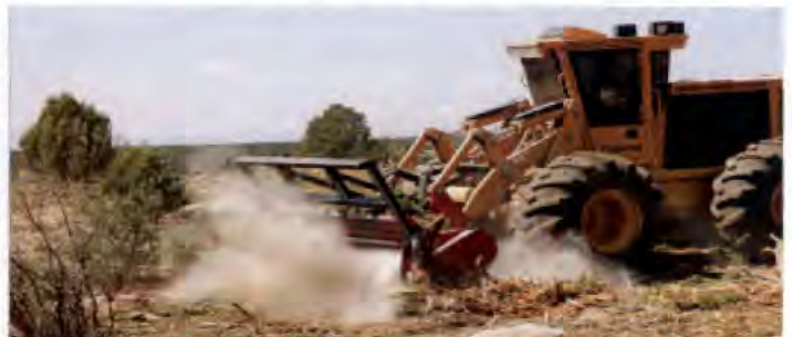
Archaeologically sensitive areas will be spared mechanized "Bullhog" deforestation like that pictured above.
