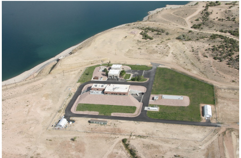
Duchesne Valley Water Treatment Plant
